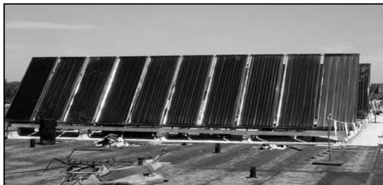
Twentyfour flat-plate 4' x 10' Collectors
