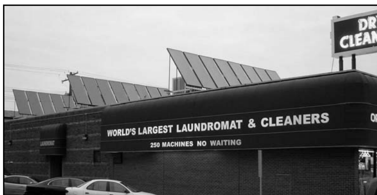
Twentyfour flat-plate 4' x 10' Collectors
