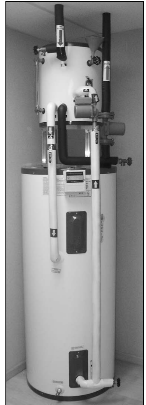
Center Picture above: The heart of a drainback system - the copper insulated reservoir tank stores the unpressurized water from the collectors that "drains back" whenever the pump shuts off. The pump should be 3' installed vertical, below the reservoir to prevent cavitation.
